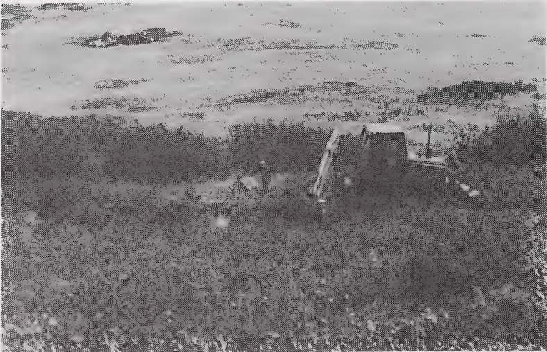
Figure 66: Backhoe trenching in slope deposits, Area 1.
